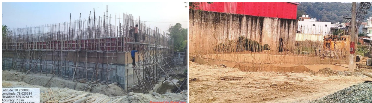
Figure: I& D Work of Rispana and STP work at Sapera Basti
