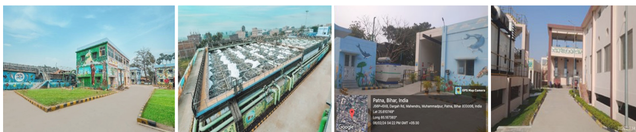
Figures: 43 MLD Beur STP, 37 MLD Karmalichak STP, Saidpur Sewerage Network, 60 MLD Pahari STP
