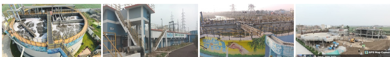
Figures: 17 MLD Begusarai STP & Sewerage Network, 11MLD Barh STP and I&D work, 8 MLD Mokama STP and I&D work, 9 MLD Naugachia STP and I&D work
