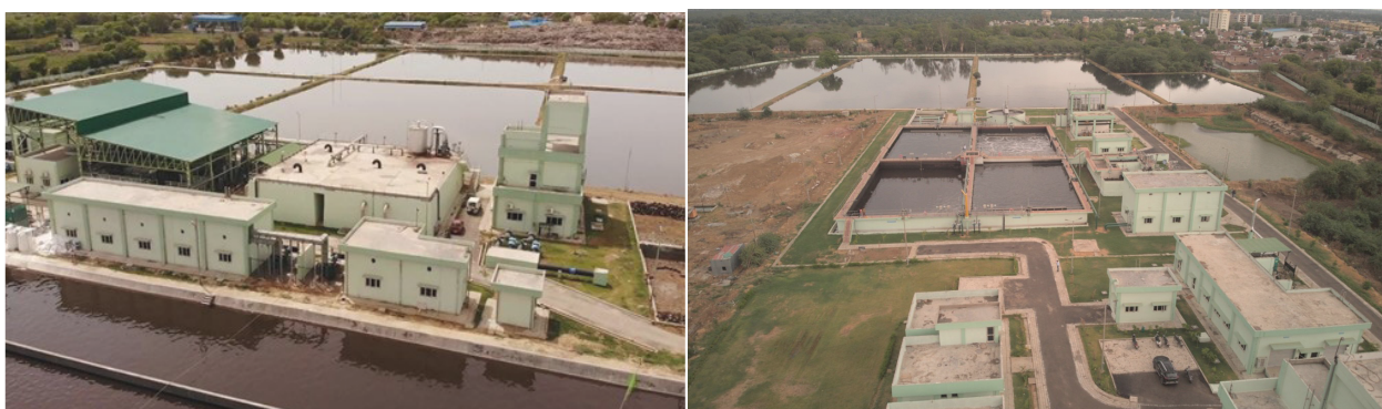
Figure: Tertiary Treatment Plant, Mathura
