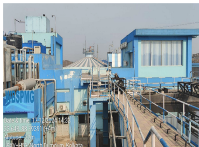
Figure: Baranagar STP
