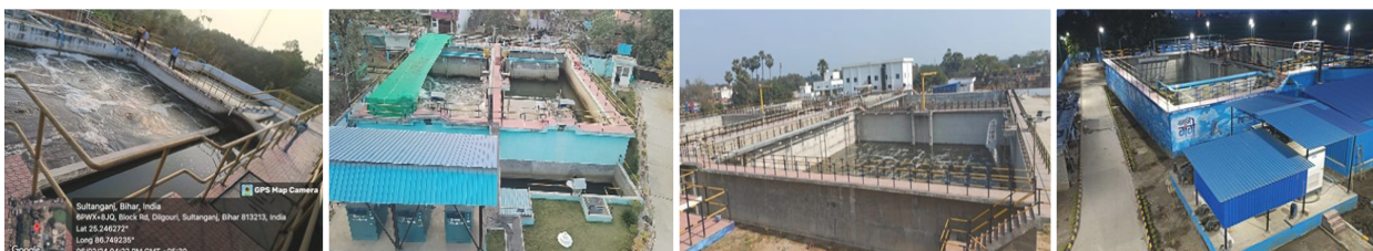
Figures: 10 MLD Sultanganj STP and I&D work, 3.5 MLD Sonapur STP and I&D work, 32 MLD Chhapra STP and I&D work,
